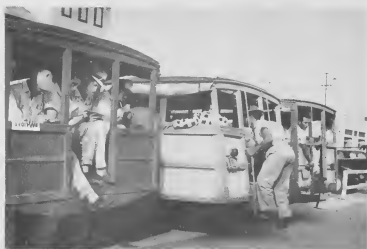
THESE TRUCKS are practically Lago land- E TRUCKAN aki practicamente ta marcanan marks. Each one can carry up to 22 men; they di Lago. Cada un por hiba 22 homber; nan ta are simply truck bodies with seats and a roof simple carga di truck cu un esaki y un dak built on the beds. They are practically indis- trahá ariba. Nan ta casi indispensable pa cien- pensable to hundreds of employees who rely on tos di empleadonan cu ta depende ariba nan them for transportation.
